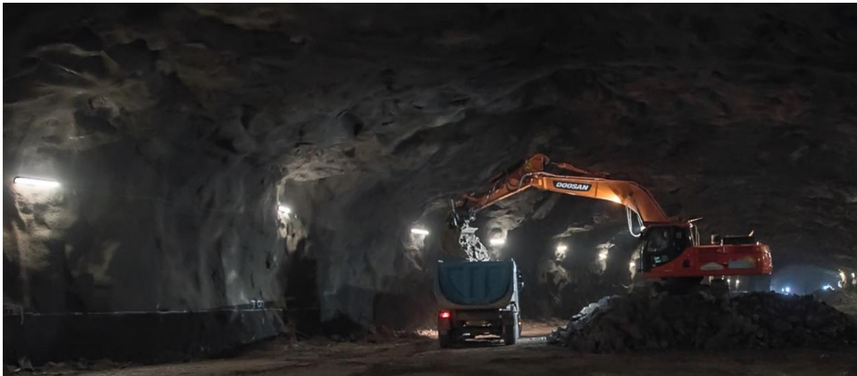
In the photograph: Länsimetro tunneling nearing completion (photo courtesy Länsimetro)
