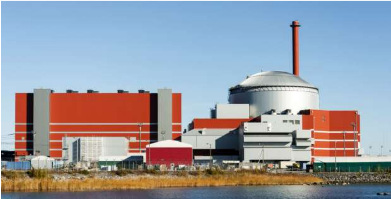
In the photograph: Olkiluoto 3 power plant as seen from the sea (photo courtesy TVO)
