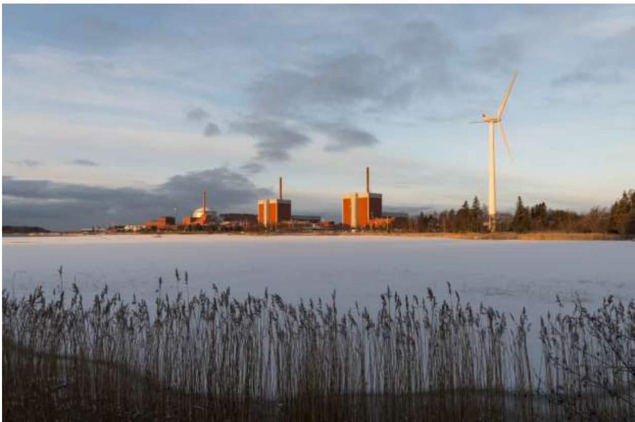
In the photograph: The TVO Olkiluoto site as viewed from the visitor center. The new Olkiluoto 3 unit is the one on the left – furthest away from camera (photo courtesy TVO).
